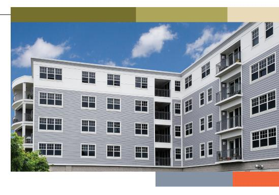
which included stripping the building back to its sheathing and installing a new adhered water-resistive barrier. Then, crews removed the previous fiber cement siding and trim, replacing it with Everlast® siding and trim over 2" of rigid insulation.
